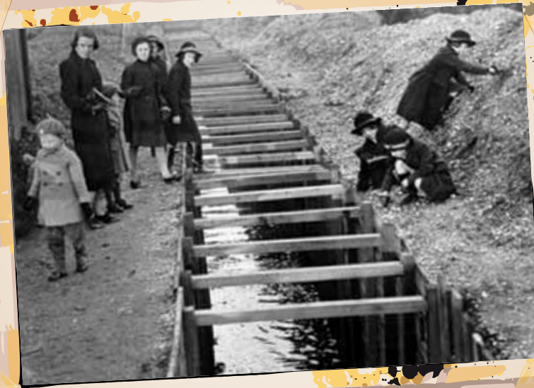
Flooded Trench, Enfield Library Green.
